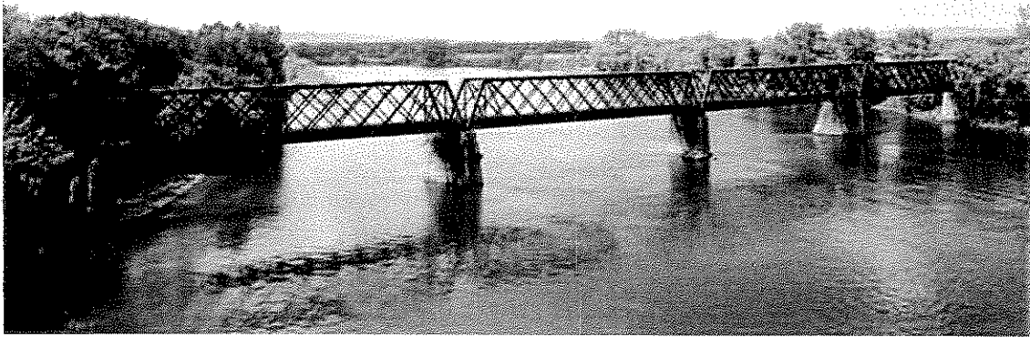
13. Boston & Maine Railroad Bridge over Connecticut River, Northampton, MA
