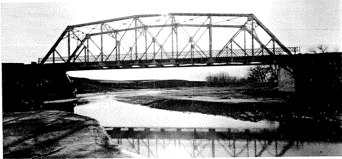
10. Cheyenne River Bridge, County Rd. 46, Niobrara County, WY
